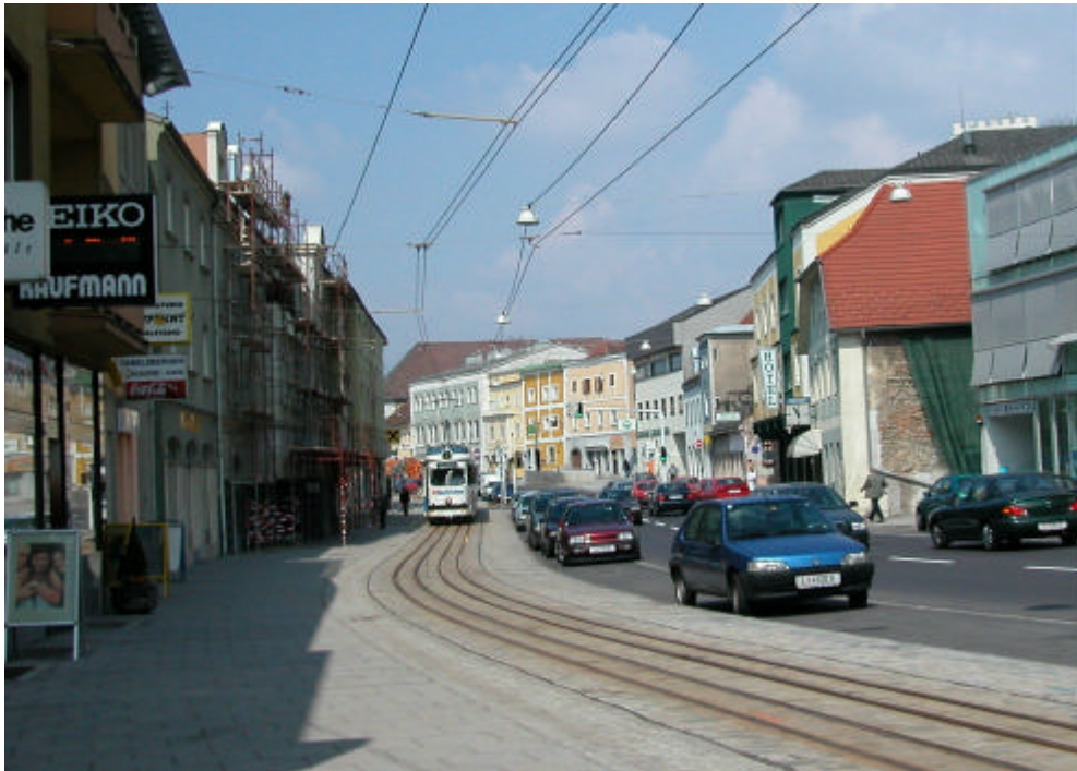
Sample LRT Right of Way adjacent to travelled lanes
