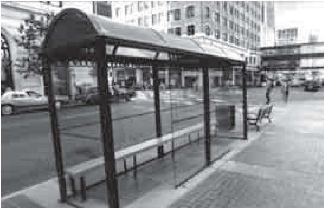
Adjacent to Alberta Treasury Branch Building, 2 Street and 8 Avenue S.W.
